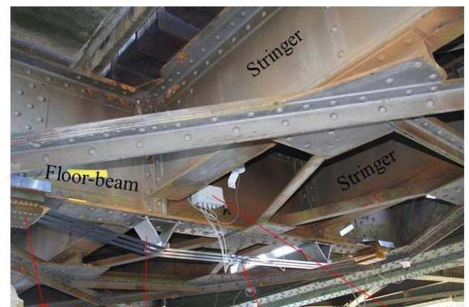
Friction clamp Column Strain gauges bonded to CFRP laminates Wireless sensor network node
